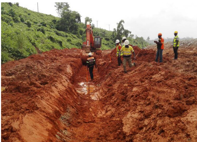
The channel was excavated, graded and shaped prior to installation
