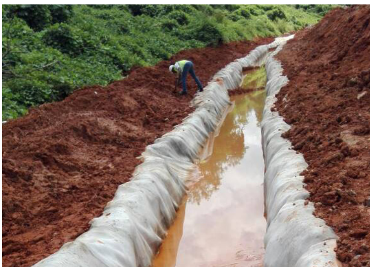
The anchor trenches were backfilled for a clean termination
