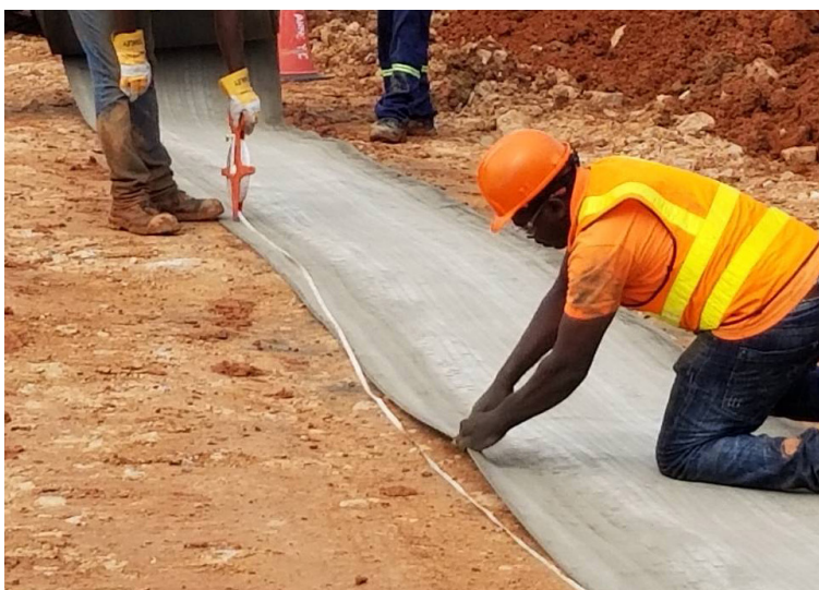
When access was restricted, CC was cut and transported to site
