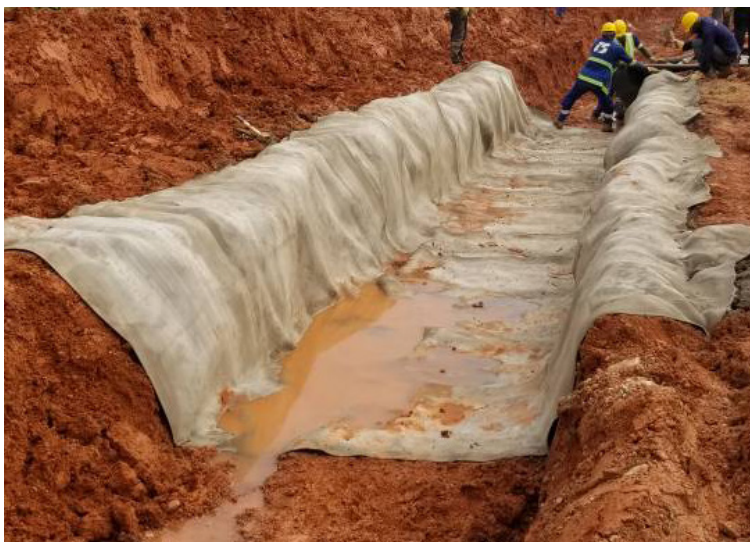
Anchor pegs were used to fix the CC into the anchor trenches and
