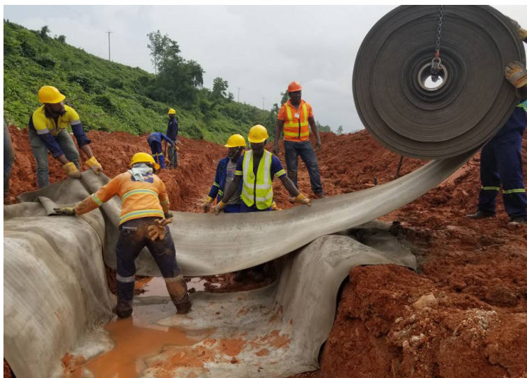
CC being unrolled and laid on site
