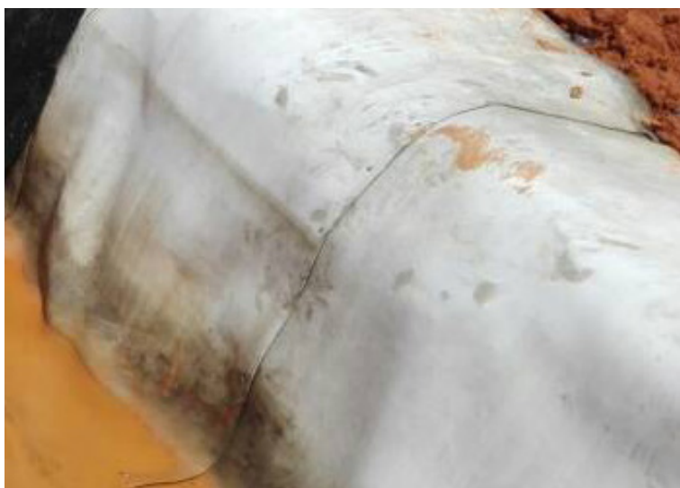
Overlaps of CC material were jointed using stainless screws
