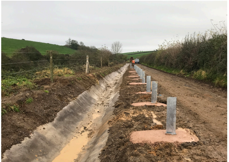
Bollards were inserted between the channel and narrow access road
