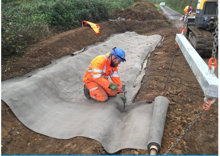
The CC was laid transversely and fixed using ground pegs and screws
