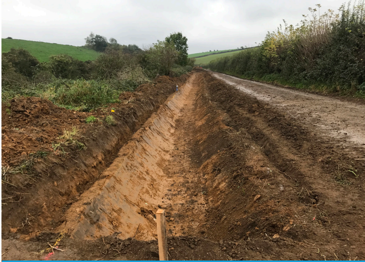
Drainage channel following excavation
