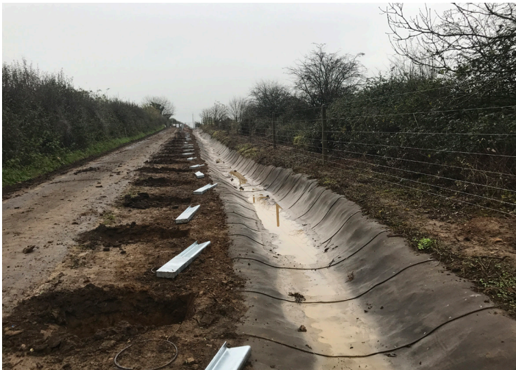
The CC edges were captured in anchor trenches and the material hydrated
