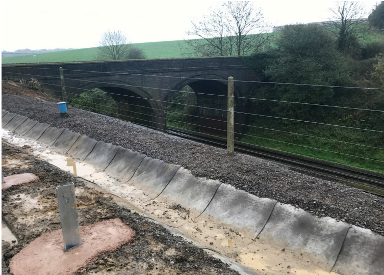
Batched rolls were used due to the channel's close proximity to the rail line
