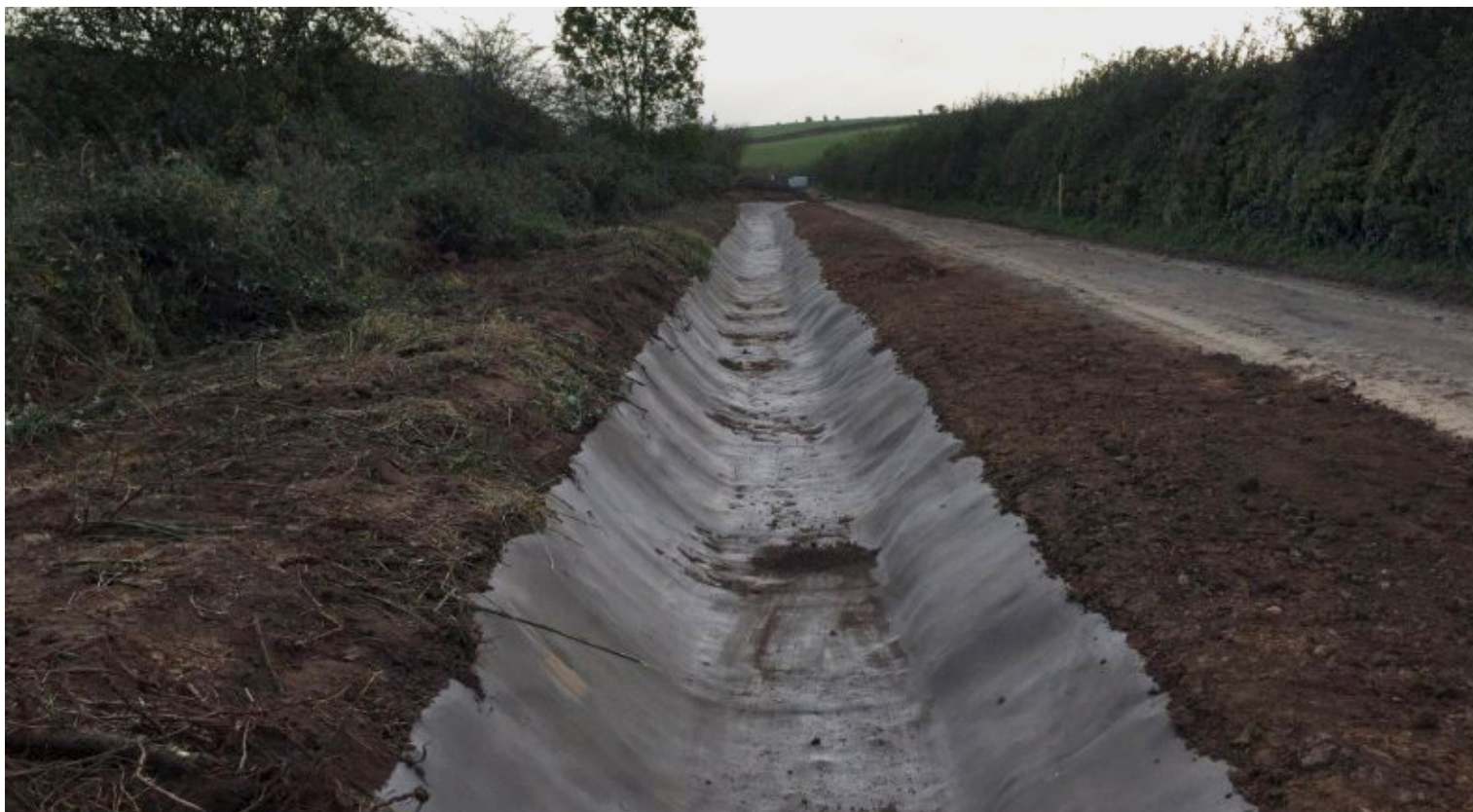
Completed section of the drainage channel
