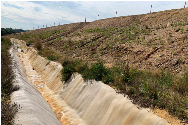
Completed perimeter channel 1 year after installation
