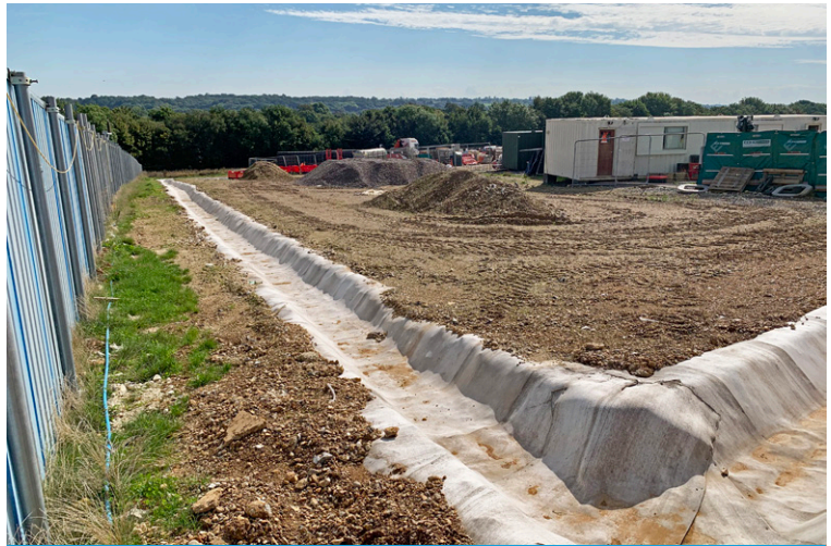
Corner detail of perimeter channel
