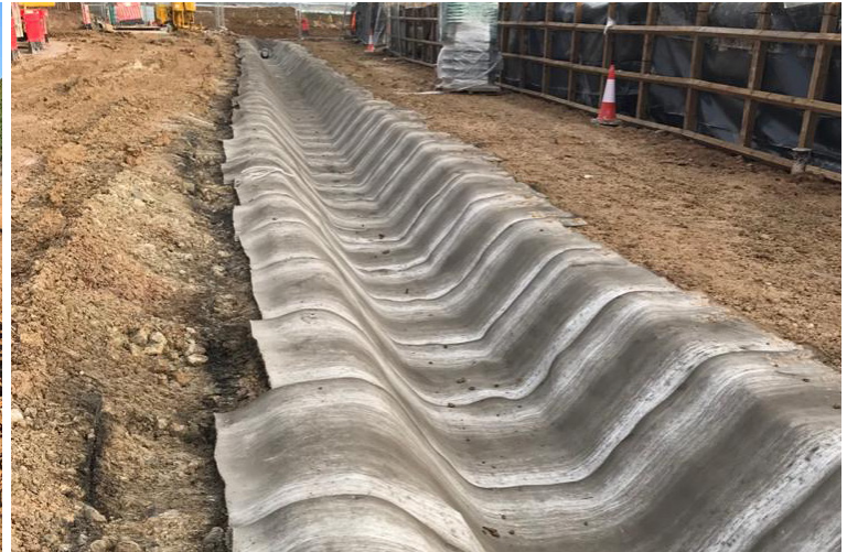
CC was laid transversely across channel profile
