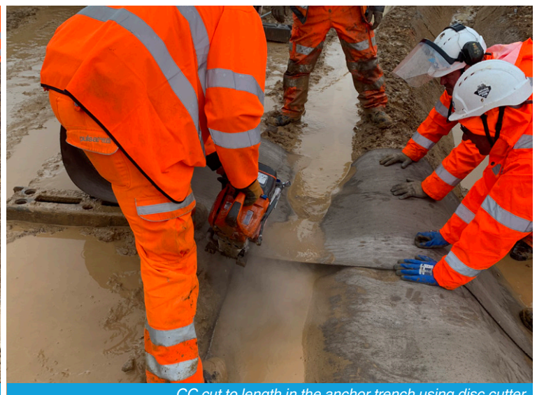
CC cut to length in the anchor trench using disc cutter
