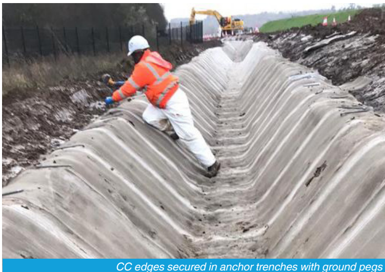
CC edges secured in anchor trenches with ground pegs
