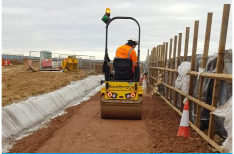
Ground on channel shoulders later compacted
