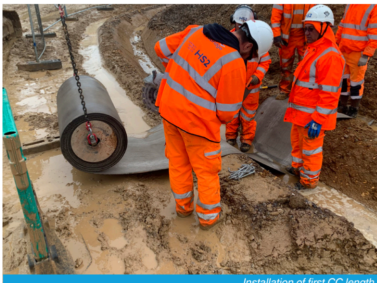
Installation of first CC length
