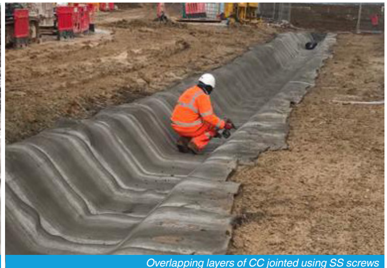
Overlapping layers of CC jointed using SS screws
