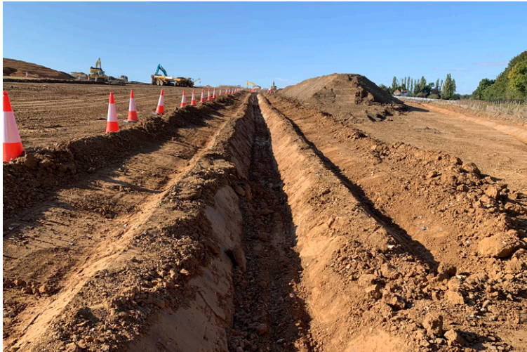
Channel was excavated using excavator with V bucket
