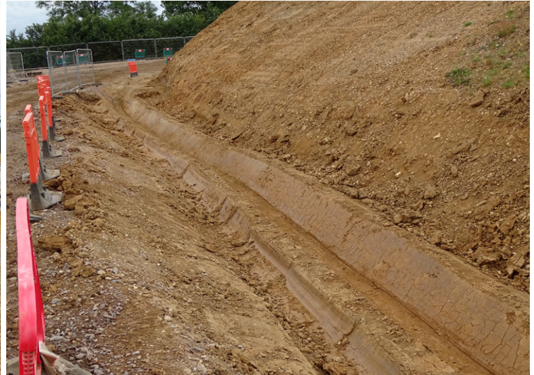
Channel profile following excavation using V bucket
