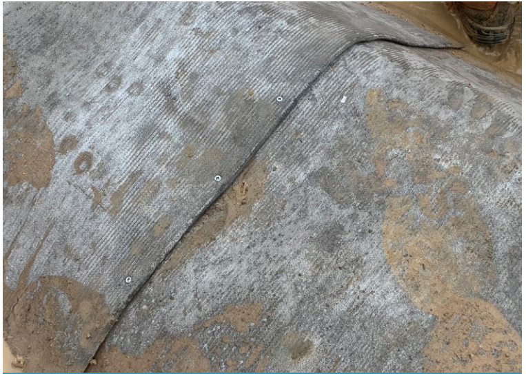
Overlapping layers of CC were joined using stainless steel screws
