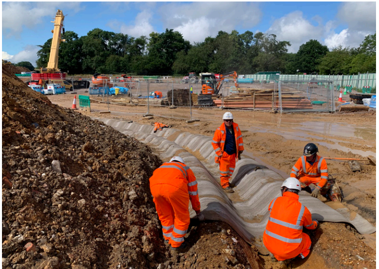
CC was able to easily accomodate bends in the channel
