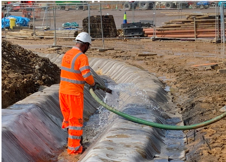
Hydration of CC using hose and bowser
