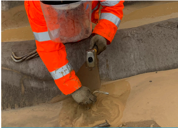
Securing CC edges in anchor trench with ground pegs
