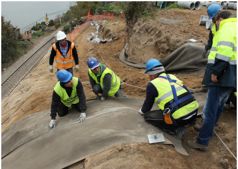
The CC layers were laid down the slope and overlapped by 100mm
