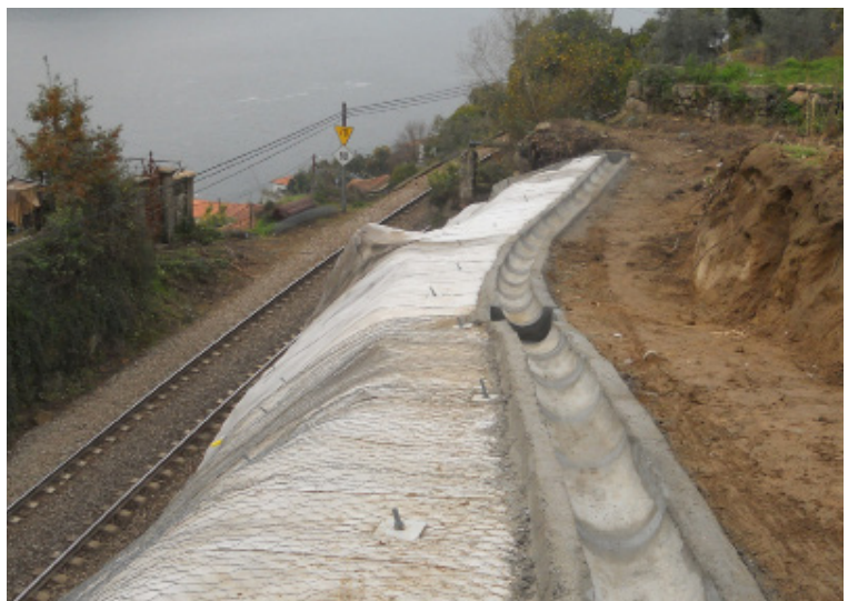
Edges at the crest were buried under a poured concrete drainage channel
