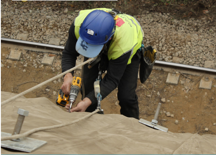
Screws were used to joint the layers together
