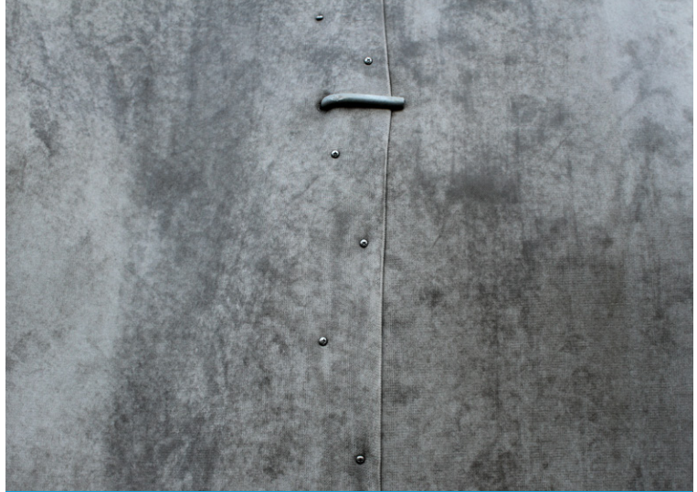
Screws were inserted in a triangular shape for greater ingress prevention
