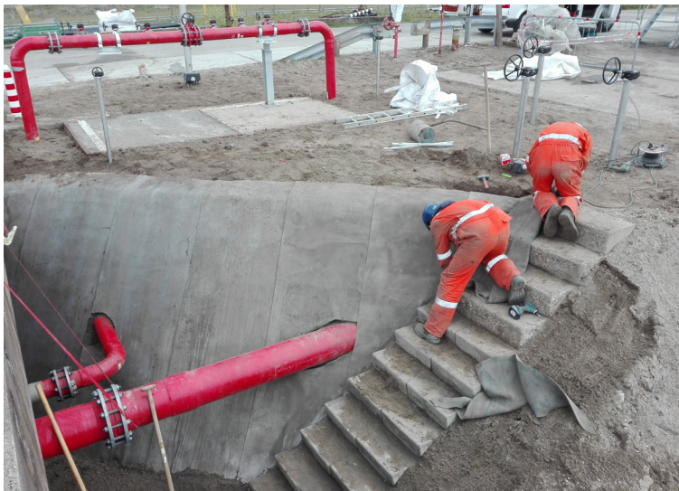
The CC was easily cut to accommodate existing infrastructure
