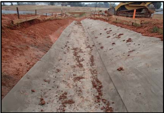
Longitudinal Panels of Concrete Cloth Deployed
