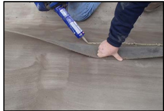
Seaming of Concrete Cloth Panels (screws added after)
