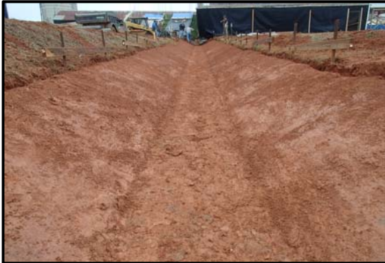
Trapezoidal Channel Prepared
