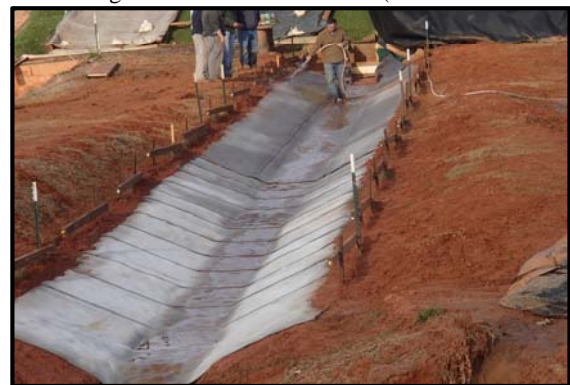
Spraying Water to Hydrate Concrete Cloth
