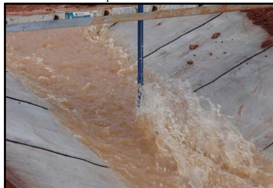
Velocity Meter Inserted into Flow
