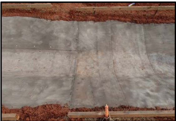
Longitudinal Panels of Concrete Cloth Meet Transverse Panels
