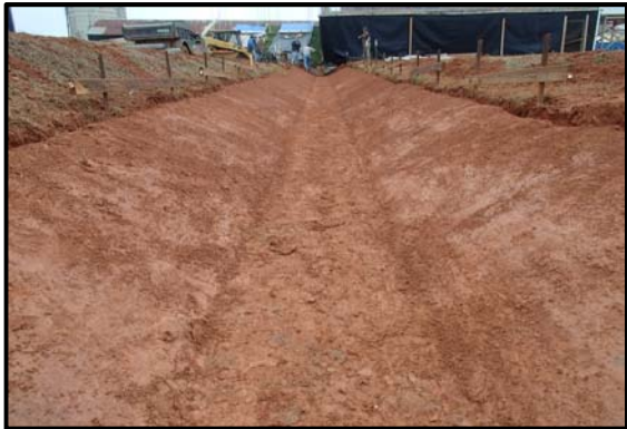
Trapezoidal Channel Prepared
