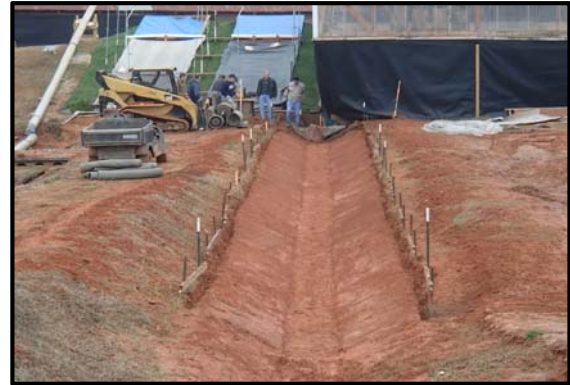
Anchor Trenches along the Top Edge of the Channel
