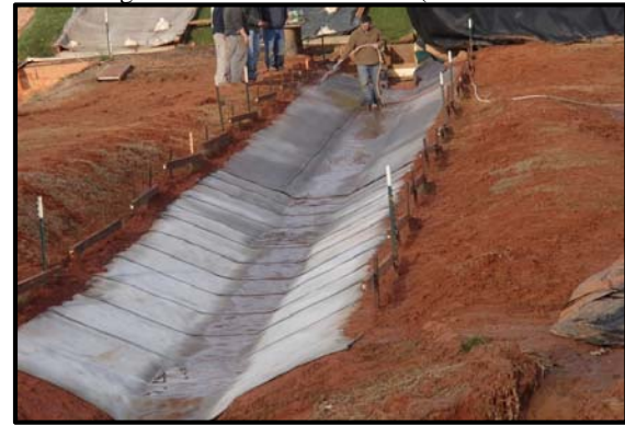
Spraying Water to Hydrate Concrete Cloth
