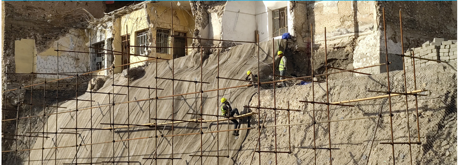
Steel mesh was installed under the CC
