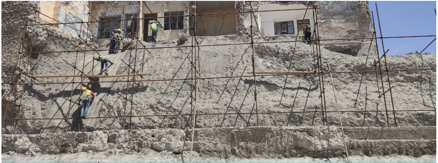
Initial stages on installation
