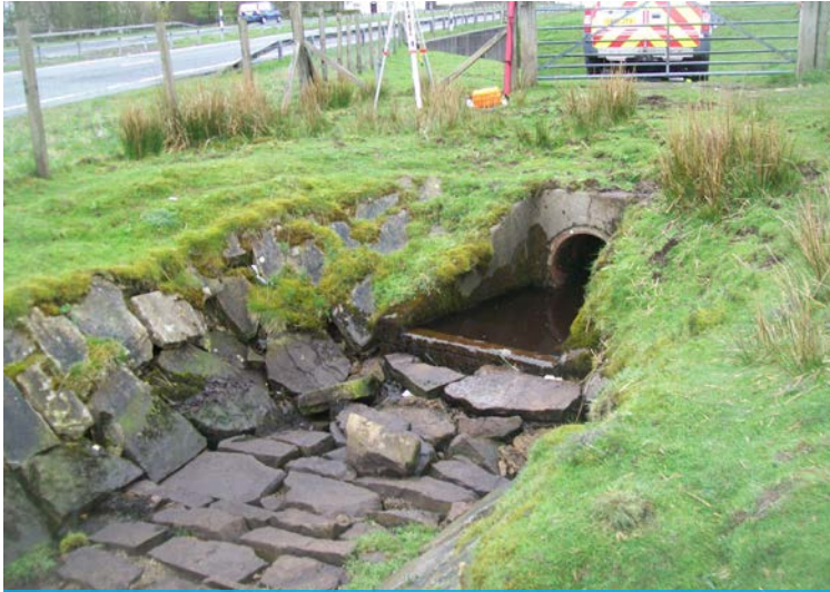
Site before works began
