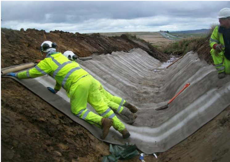
Batched CC8™ being unrolled
