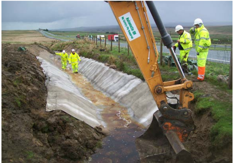
Allowing the live water course to hydrate the CC
