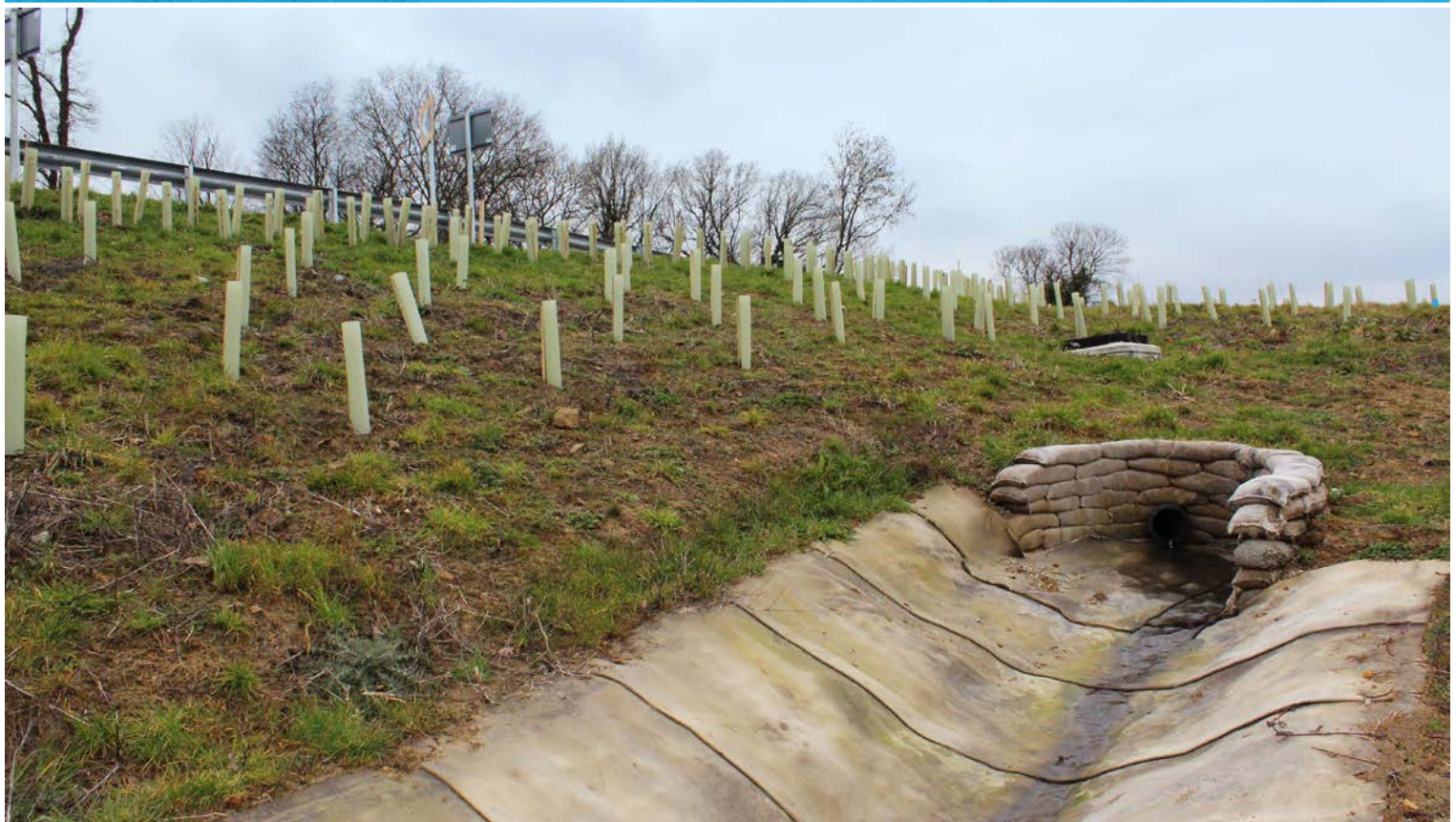
CC connected to concrete sandbag headwall
