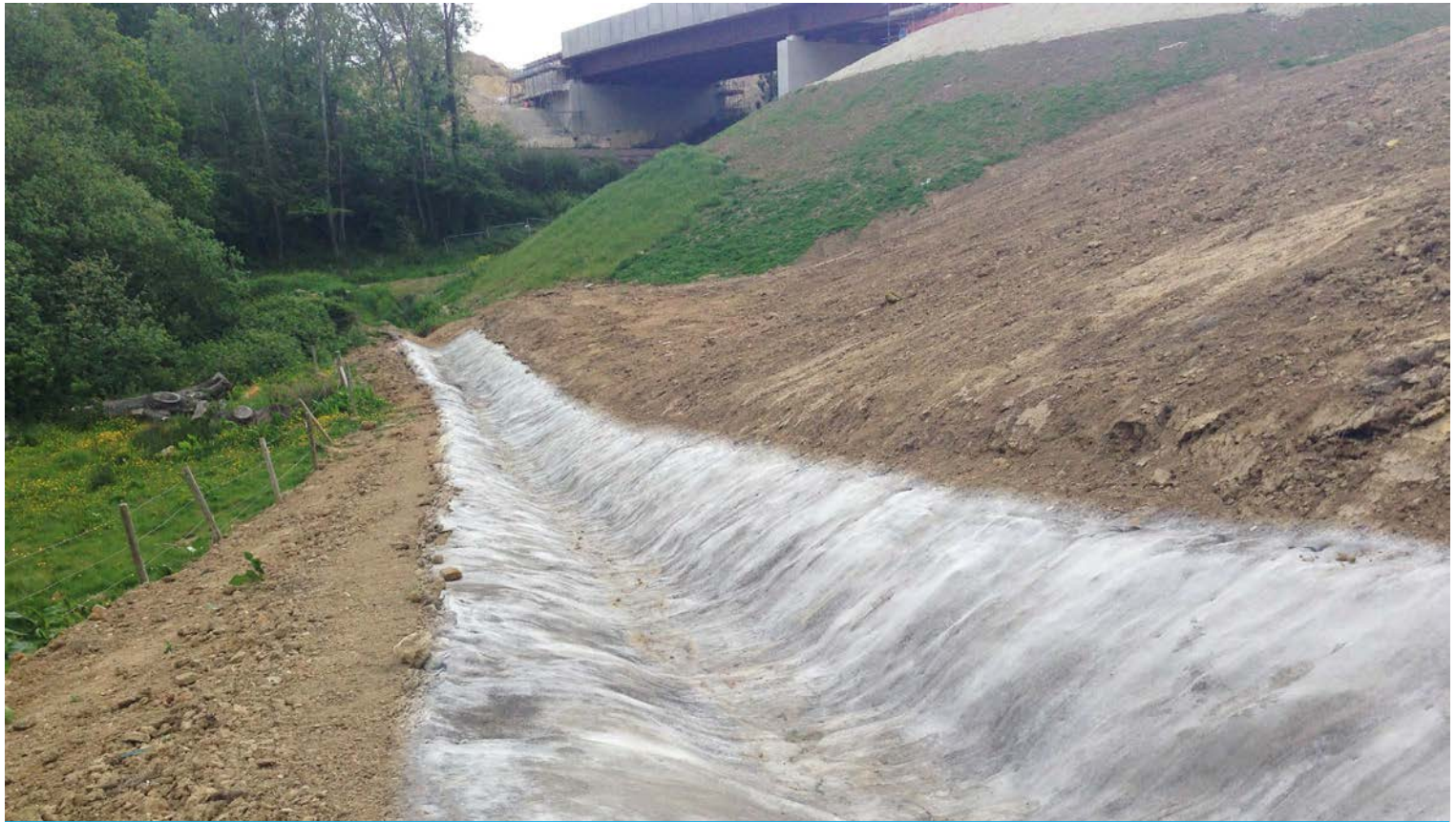
Immediately after installation
