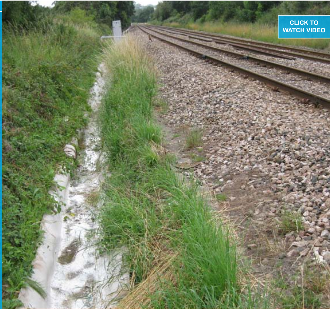
Completed lined carrier drain
