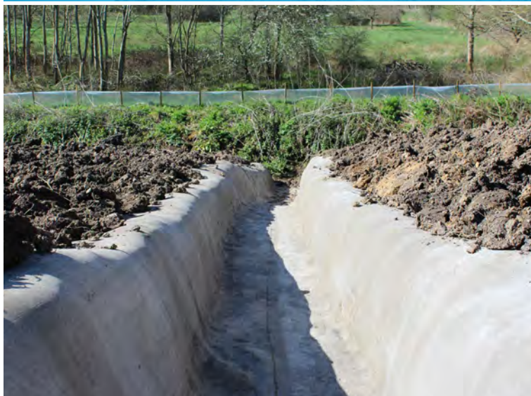
Backfilled anchor trenches
