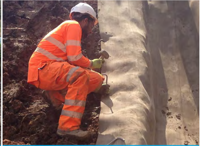
Pegging into the anchor trench
