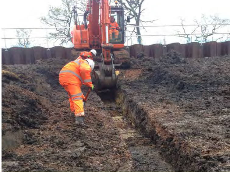
Excavating the ditch and digging a shallow anchor trench
