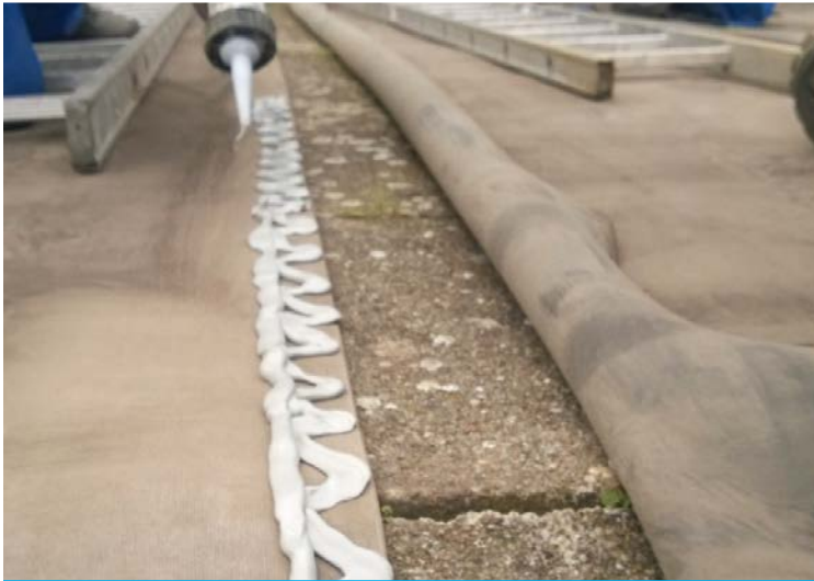
Sealing under the overlap
