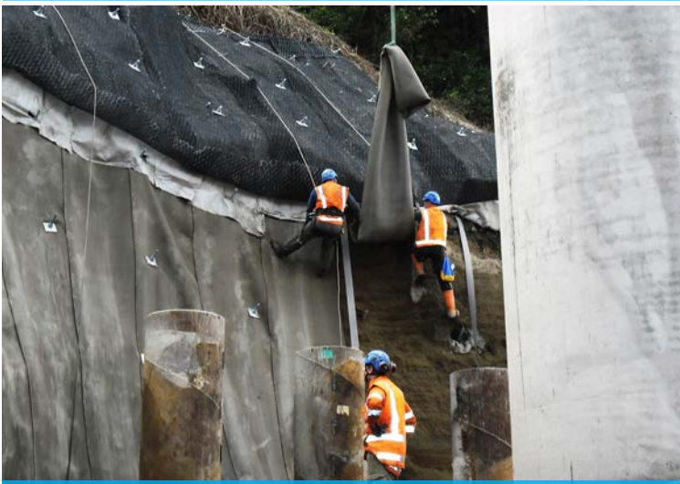
Installation under the geotextile
