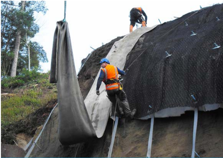
Engineering anchors pushed through the matting
