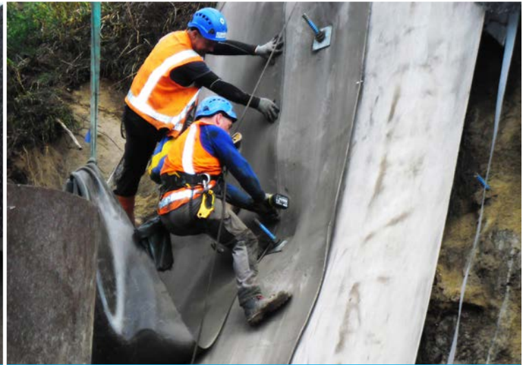
The joints being screwed
