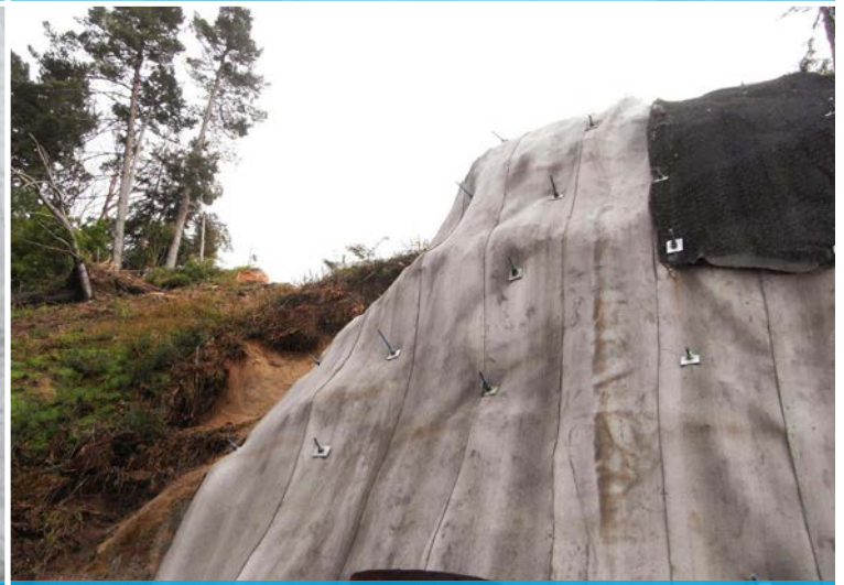
The finished installation
