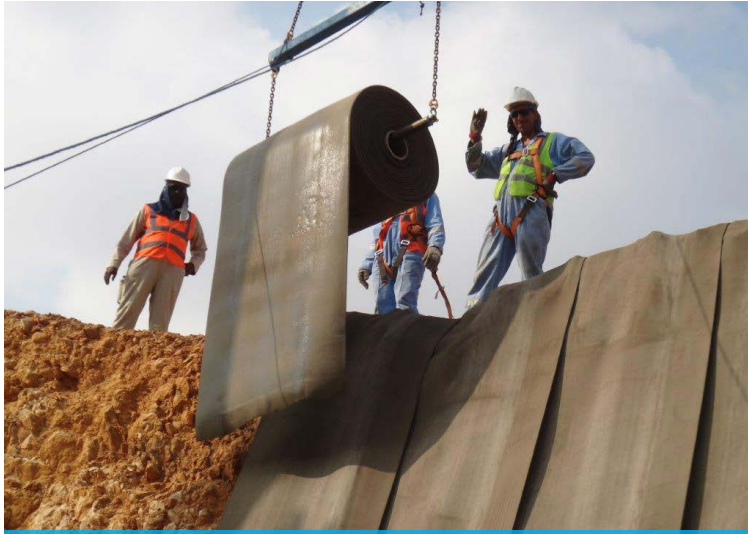
CC being lifted into position
