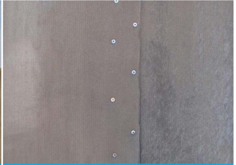
CC jointed with two offset rows of screws
